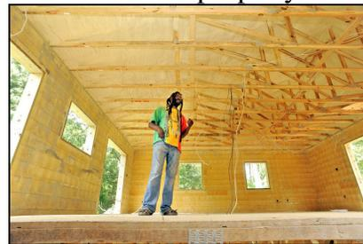
Gary Pretty stands on the second floor of his building. Above him, the ceiling has been sprayed with layers of closed-cell polyurethane foam.
