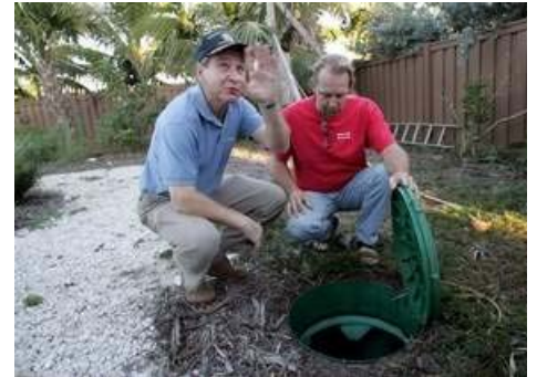
Homeowner Mark Baker, right, shows the cistern of his Indialantic home to Titusville Mayor Jim Tulley on Saturday. cistern returns runoff to the ground and not the river. (Christ Stuart, FLORIDA TODAY)
