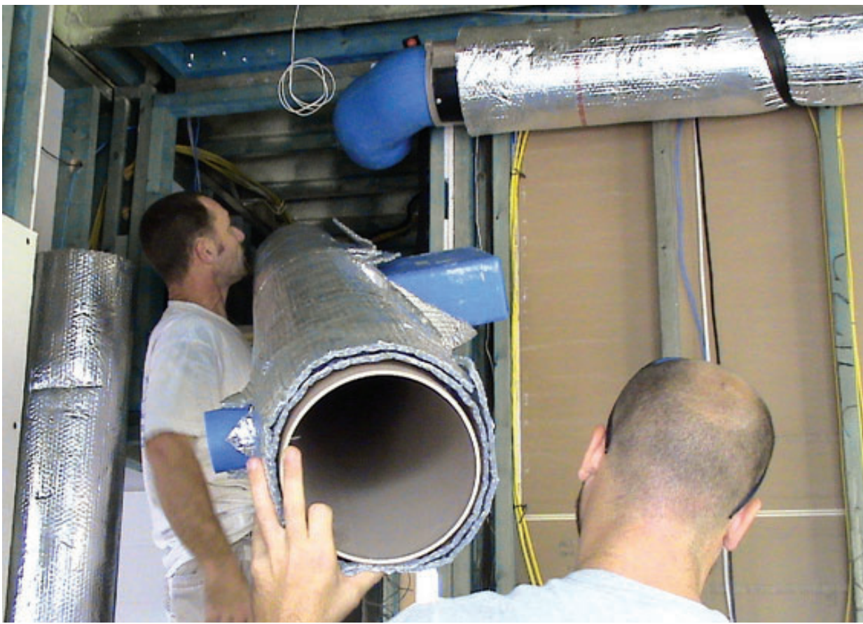
Installing the Zero-Loss Duct™ manufactured by CDC Industries
